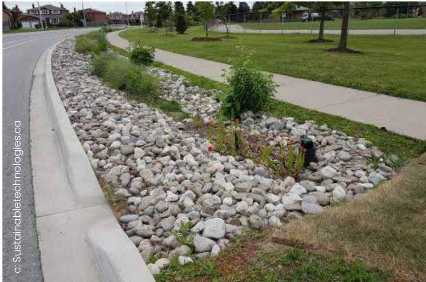
Figure 4.67. Bio-swale at County Court Boulevard, Brampton.
