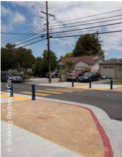
Figure 4.54. Introduce curb extensions at all intersections where a permanent parking lane exists to increase sight lines between pedestrians and drivers.
