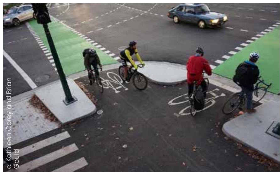
Figure 3.15. Protected intersections increase driver visibility of people in the crossbike and crosswalk by setting back the crossbike from the motor vehicle travel lane.
