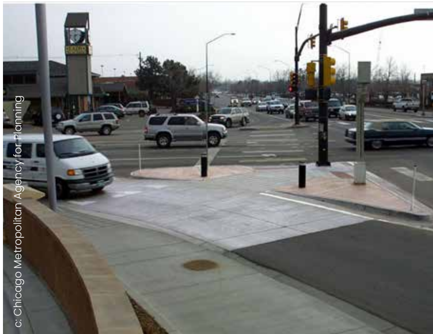
Figure 4.56. A tabletop pedestrian crossing in an existing slip lane permits turning but reduces speed and improves accessibility and visibility of vulnerable users.
