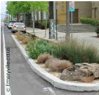
Figure 4.36. Curb extensions in a parking lane provide additional greening and stormwater management opportunities.
