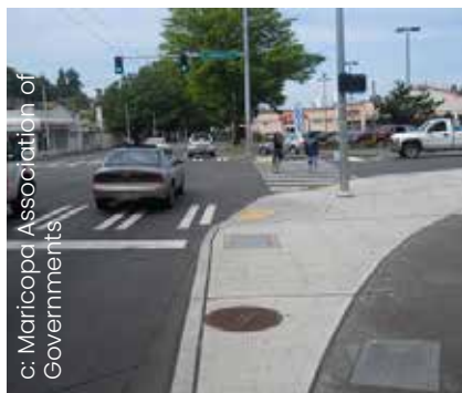
Figure 4.44. Smaller curb radii shorten crossing distances and reduce vehicle turning speeds (Seattle, WA).
